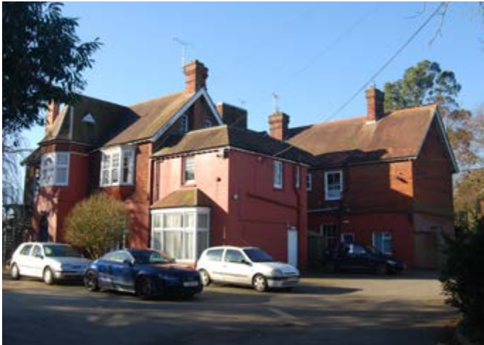
Photo 120: Ladymead, formerly Hurstpierpoint Grange
