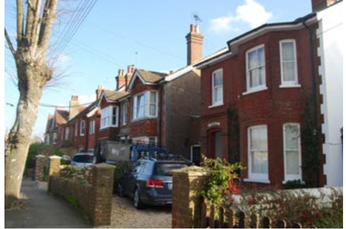
Photo 103: Front garden walls on South Avenue
