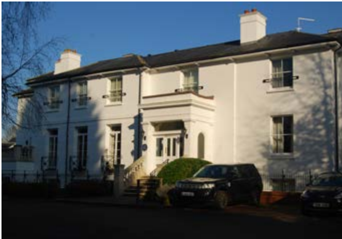
Photo 88: St George's House
