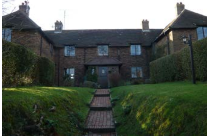
Photos 140 and 141: Arts and Crafts terrace at 16-20 College Lane
