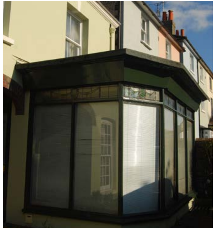
Photo 40: The shopfront at 17 High Street
